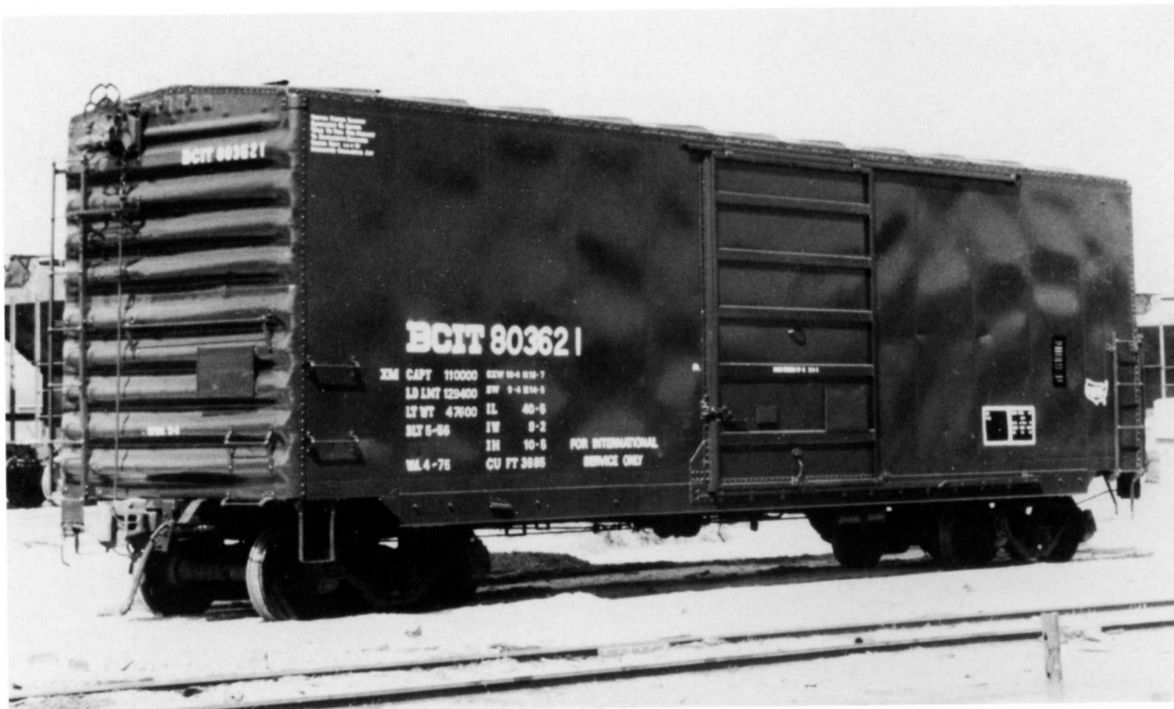
TOP Here is another cream-colored rebuild. Part of lot 1266, there were 150 of these "reconstructed boxes" built in April 1974. ATW 6105 was originally built in March 1954. These cars were "XF" classed and assigned to the Buffalo Creek Railroad at Buffalo NY. This series was
