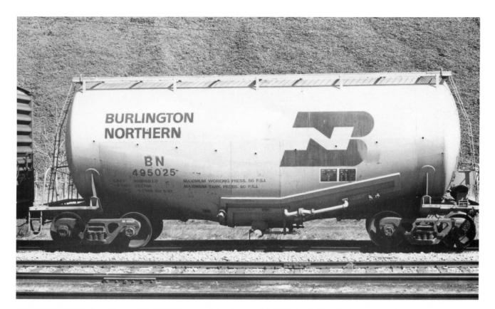
GATX 207A60W design (above). BN 495025 is essentially the same type of car as the Baroid car. This one is rated at 2,800 cubic-foot, too. Series, BN 495000-495049 (CB&Q 84950-84999). Outside length, 41'3".
