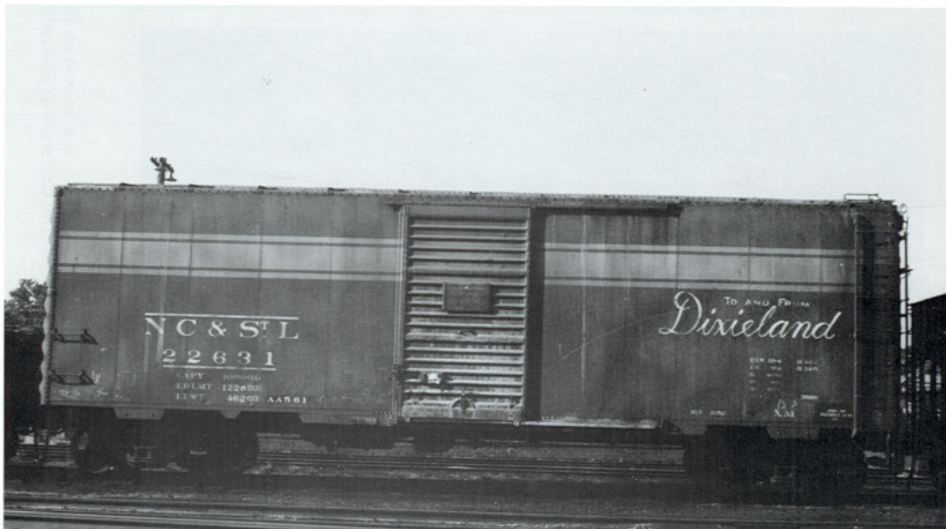
These two cars illustrate the paint scheme worn by the NC's boxcars to the end of the Railroads' days. Both cars are out of the 22000-22649 series, built at Pullman-Standard in 1952. 642 cars survived to be transferred to the L&N 13950-14592 number series. Both of these cars were photographed by Paul Dunn around 1960-61, locations unknown. both photos courtesy Rich Burg
