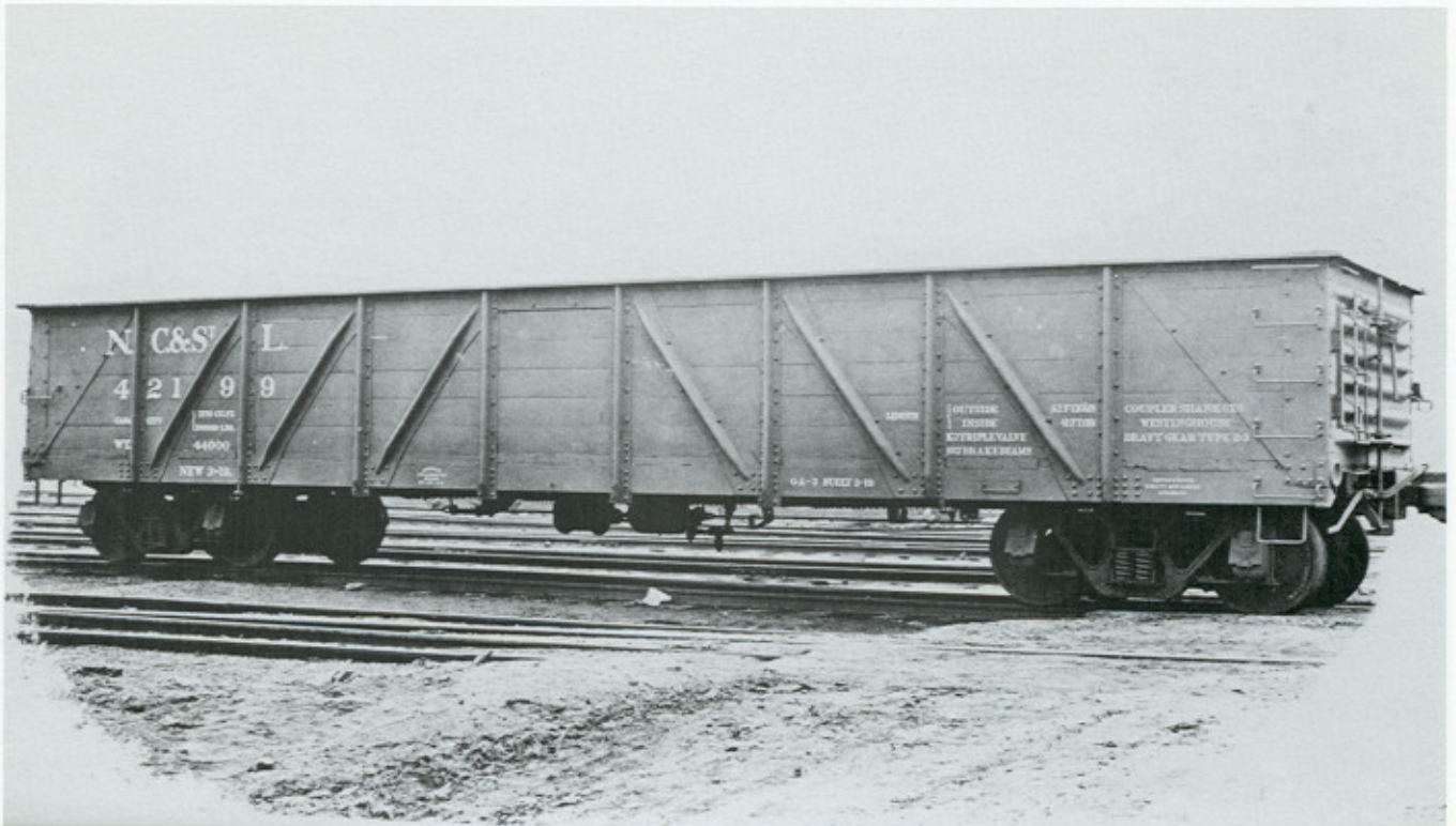
TOP: A group of cars from the GA-3 class, these cars are apparently being rebuilt, based on their incomplete stencilling. This photograph, taken at the NC's Nashville shops in 1926, illustrates a quite unusual type of car: note the wooden upper sides, along with the splice plate situated in the middle of the lower, steel sides. This car, originally built 10-13, probably entered into coal service. photo courtesy The University of Louisville BOTTOM: NC 42199 shows off more conventional lines in her ACF builder's portrait, taken in 1919. Most interestingly, these cars are ALSO marked as GA-3 class. Just why such two totally different car designs should have the same class rating is quite confusing, though an explanation probably did exist at the time. photo courtesy Ed Hawkins and ACF
