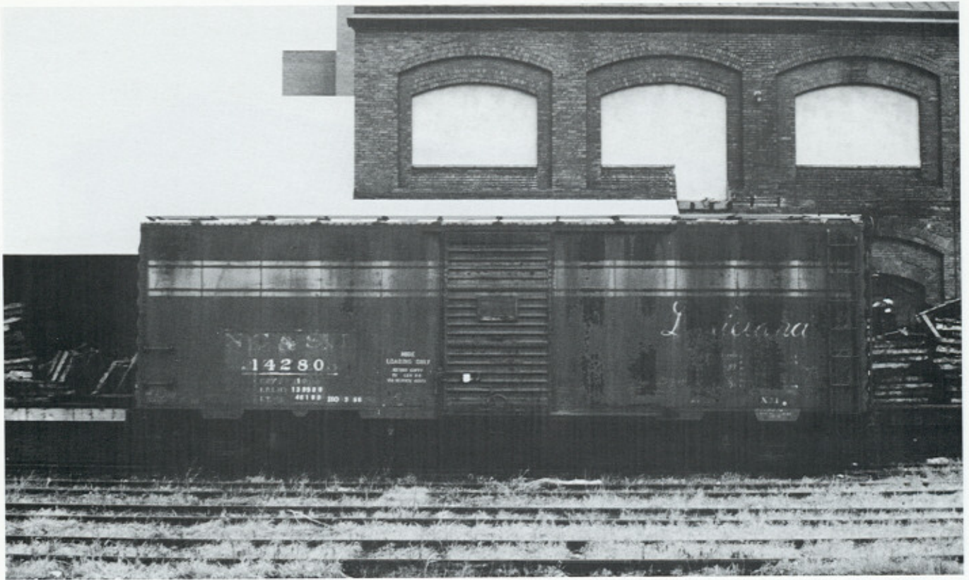
TOP: When stencilled "Hide Service", it can be assumed that the car bearing the stencil is nearing the end of it's useful life. L&N 14280 is originally out of the NC series 22000-22649, built at Pullman-Standard in 1952. This car was spotted at Reading, PA., far from it's assigned territory on the L&N. photo courtesy C.T. Bossler. BOTTOM: NC 46684 has obviously seen better days when here photograph was taken at Willow Run, MI. in March 1978. One of the few cars to still sport its original marks and number at that date, it also acquired an ACI label. photo courtesy Rich Burg
