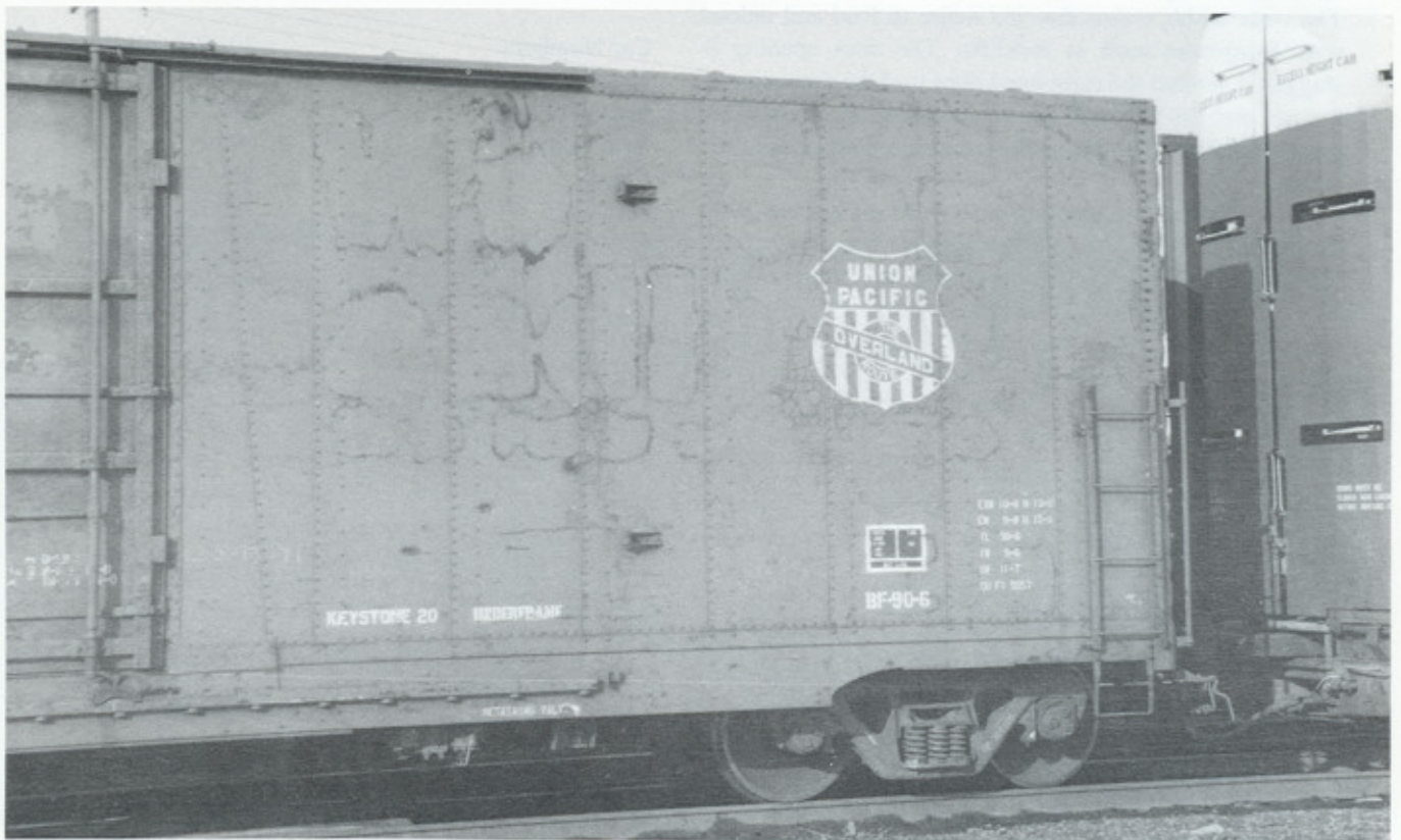
(Above) A view of the left side of the car, showing the simple, white lettering that has been stenciled on the brown paint. Note the Plate E clearance notice to the right of the car number. Only the light weight and load limit of the car are given. (Below) A view of the right side of the car, showing the Union Pacific shield, with the car class and dimensions below it. Judging from the peeling paint, the "We Can Handle It" slogan and a larger UP shield were once on the side of the car.
