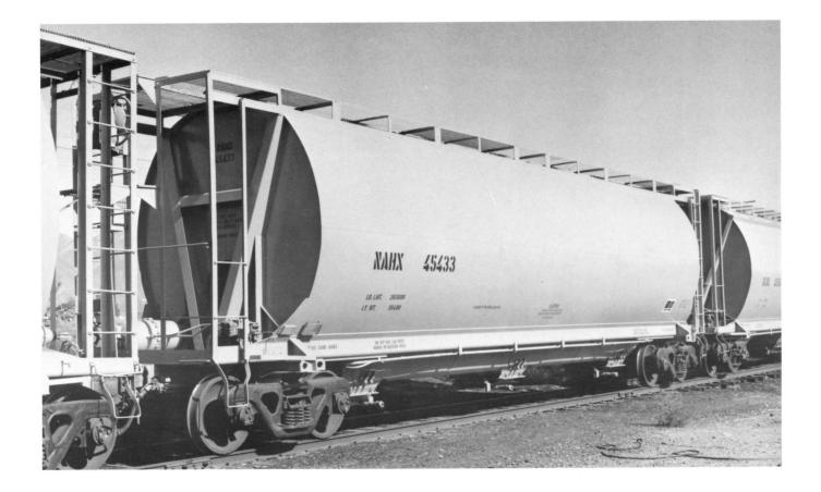
(Above) NAHX 45433. Built 11-66. 3500 cu ft capacity. TG Soda Ash lessee. Salt Lake City, UT, 8-92. (Below) NCHX 45661. Built 4-67. TG Soda Ash lessee. Salt Lake City, UT, August 1992.
