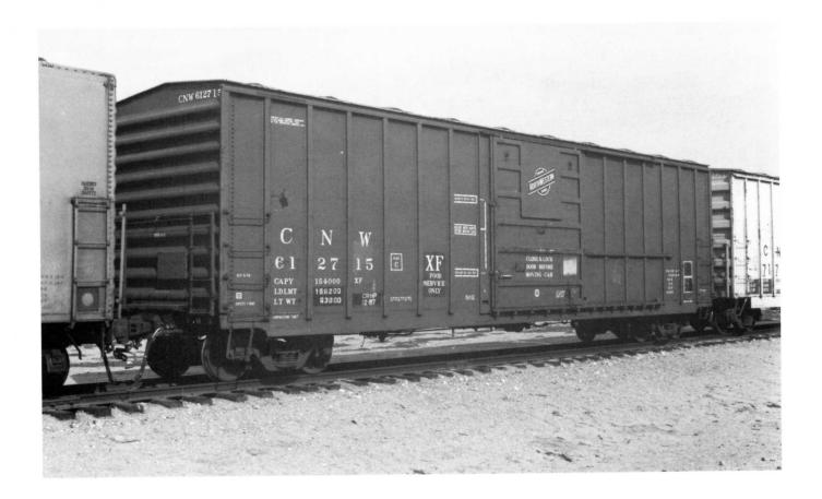
(Above) CNW 612715. 154 XF. 5277 cu ft capacity. ex-NSL. Built 5-78 BFF RV. CNW 612700-612787. (Below) CR 361103. NYC lot 936B. Built 10-64. 4678 cu ft capacity. 140RBL.
