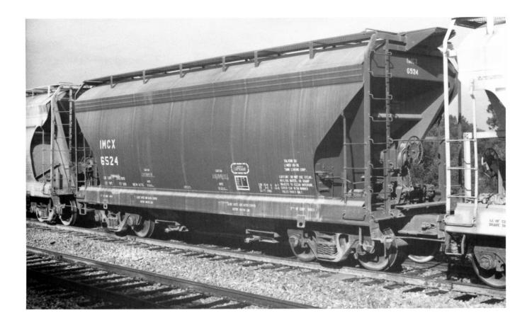
(Above) IMCX 6524. Built 8-78 ACF MILT. 2980 cu ft capacity. Lined Talicor 50 10-78 by TLC. (Below) KCS 756156. 188XM. Itel owner-lessor. nee-PW. Built in 1978 by ACF STL. 6685 cu ft capacity.
