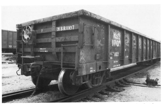
(Above) NSR 11107, "B" end view. Of particular note are the vertical stiffeners which are bent in at the bottom. Also note the heavy demarcation line between the car side and the lower side channel. (Below) NSR 11107, "A" end view. Of particular note here is how the 6"x6" top chords project out past the car ends. Note also the "2240" cuft capacity markings. Both photos by James Kinkaid.
