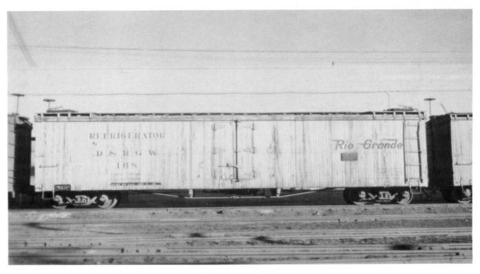
Above. DRGW 168. Narrow gauge reefer. Courtesy R.W.Richardson. Below. C&S 1105, narrow gauge refrigerator car at Denver, Co on July 30, 1938. Richard H. Kindig.
