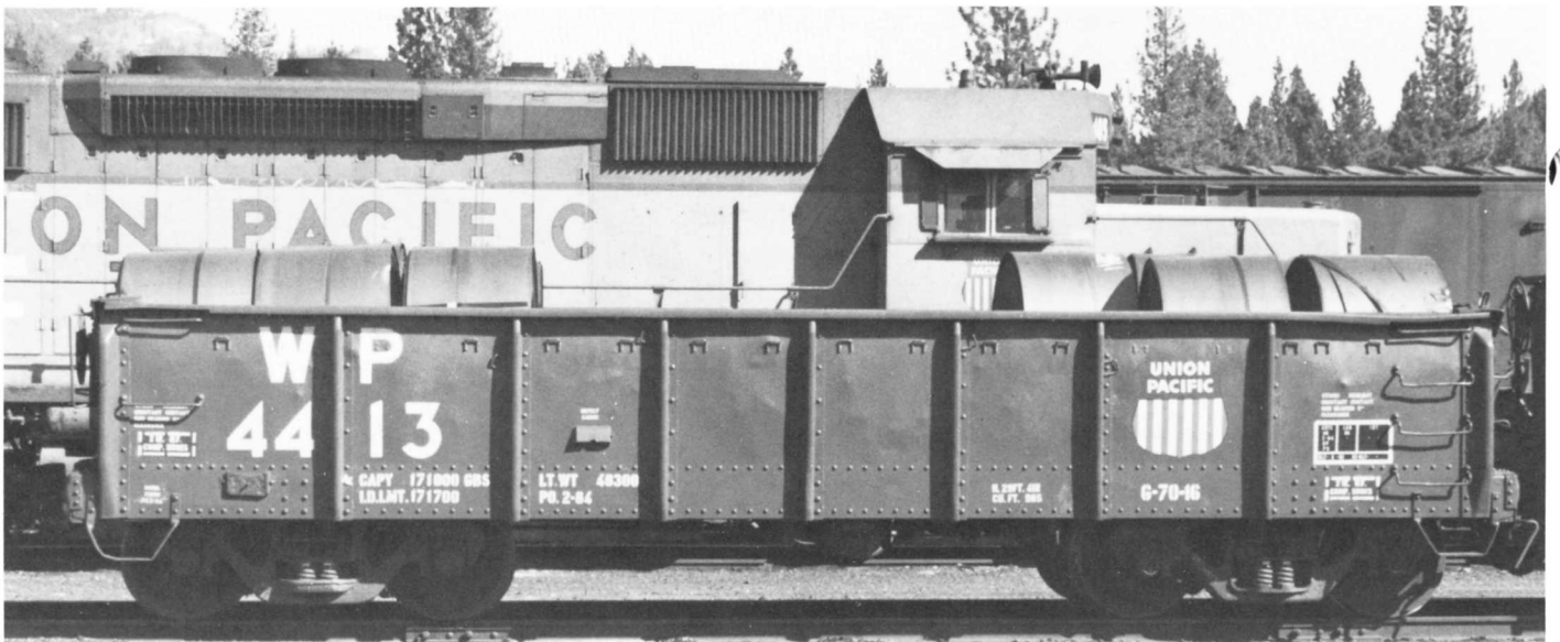
Greenville built these shorty (29') Gonds for coil steel service.
