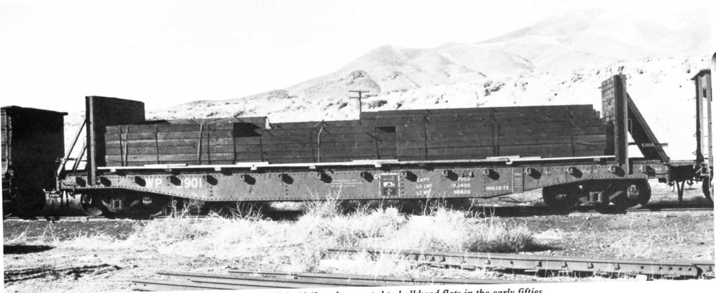
These flat cars were BLT in 1942 and converted to bulkhead flats in the early fifties.
