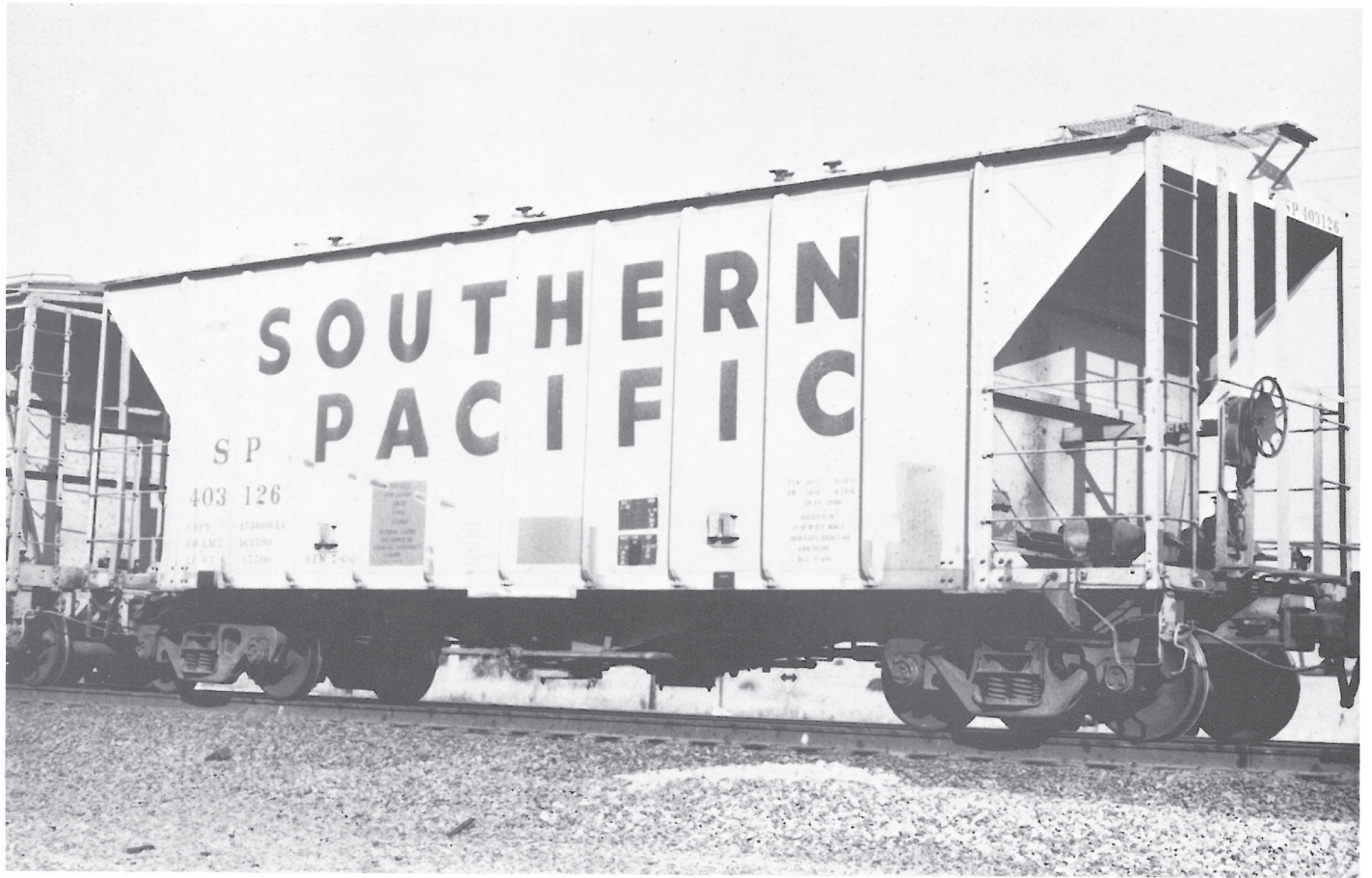
SP 403126. A single bay GATX "Airslide" built in 7-68.
