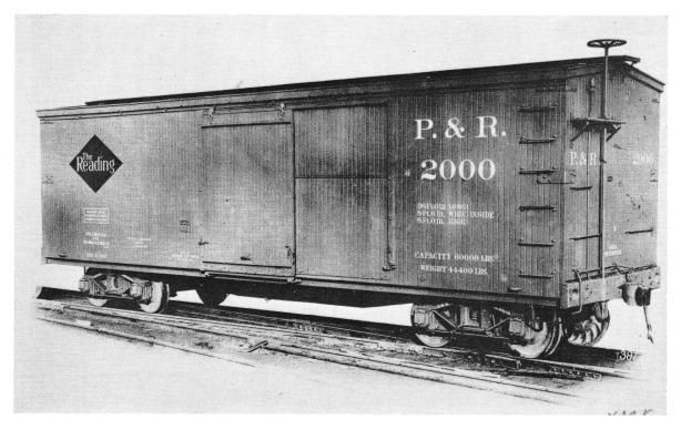
P&R 2000 is part of a series of 1000 cars built 1907-08 by the Standard Steel Car Co.
