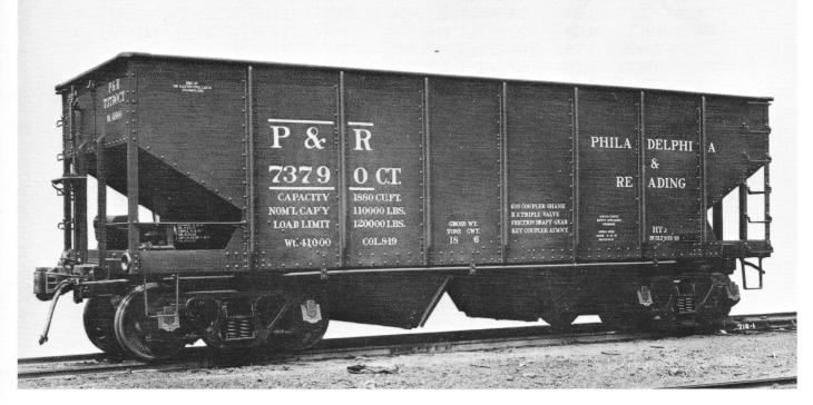
P&R 73790, class HTJ was built 8-12-19 by the Ralston Steel Car Co. at Columbus, Ohio. Note the cubic capacity is the same (1880 cuft) as the Standard Steel built P&R 77004.
