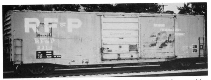
(Above) RF&P 2310 shown here in San Luis Obispo on 4-5-86 was built by Pullman-Standard in 1963. The car was scaled on the Seaboard System in 6-85. Door is aluminum, white lettering, data, logo. Light weight and capacity area was painted black after being scaled. Pat Holden photo
